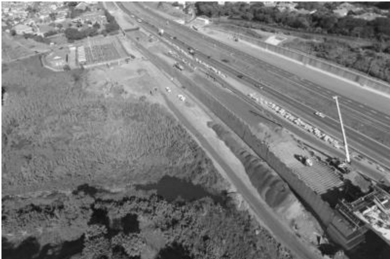
Figure 2. Aerial photograph of MSE Walls 6 and 7
