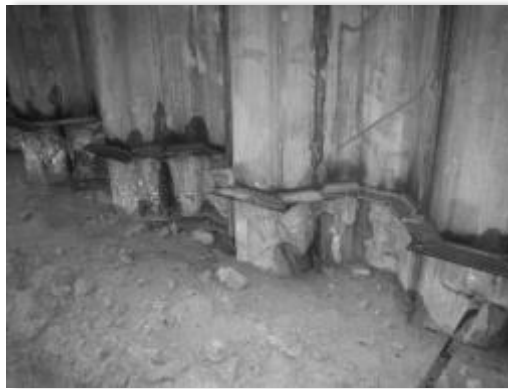
Figure 11. Welded interlocks inside basement to ensure water tightness.
