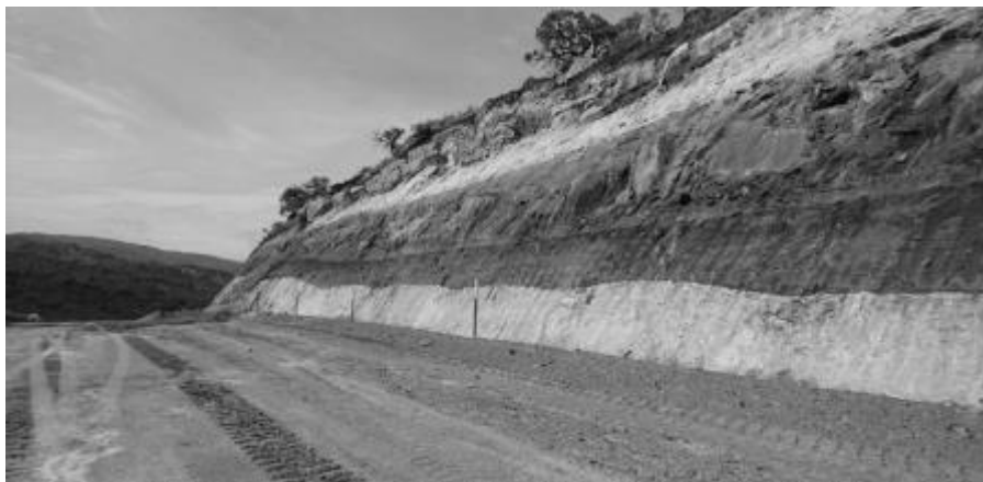
Figure 3. Cutting on access road excavated to some 10m deep
