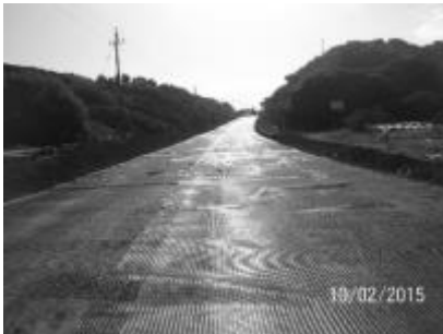
Figure 9. a) During construction
