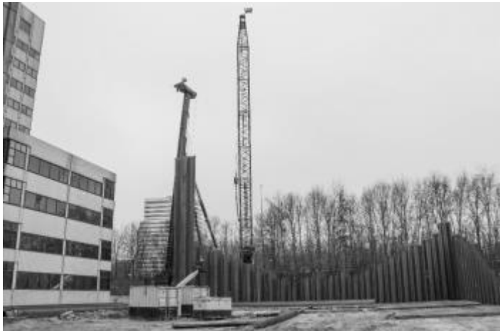
Figure 6. Phase 1 – Installation of Sheet Piles
