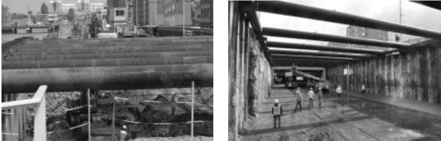
Figure 12. Tunnel construction in Neherkade, Den Haag, Netherlands
