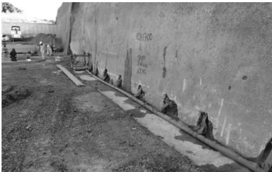
Figure 5. Drainage of layerworks and temporary soil nail wall band drains
