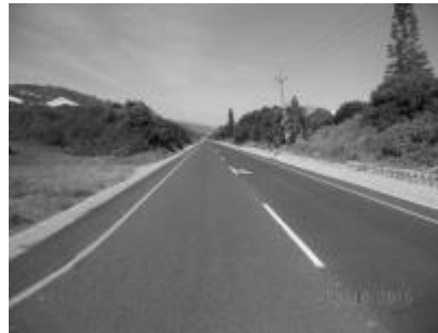
Figure 9. b) Completed project
