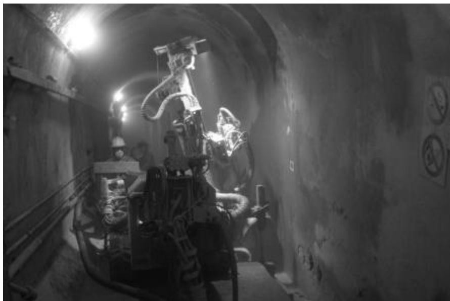
Figure 4. Drilling operation inside the drainage gallery
