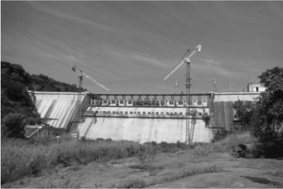
Figure 1. View of the Hazelmere Dam during raising
