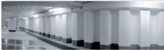
Figure 10. Basement Parking - Sheetpiles
