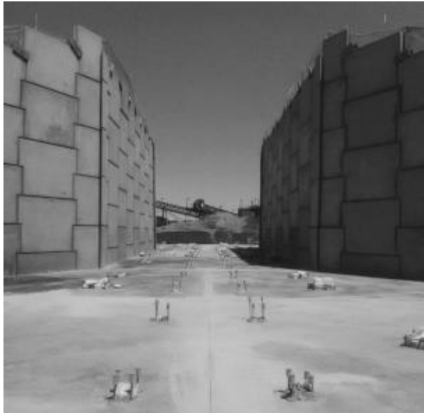
Figure 3. Two of the Four Completed Walls
