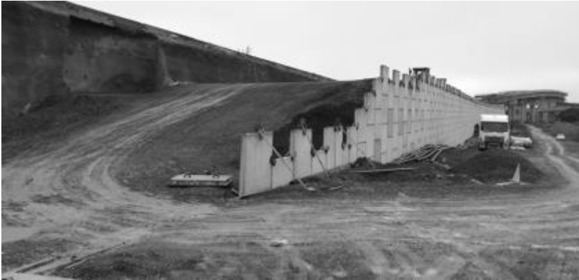
Figure 7. Bottom access ramp between MSE Wall 6 and Mount Edgecombe Drive Underpass
