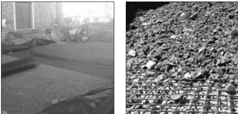
Figure 6. Construction of the geosynthetic reinforced soil raft foundation
