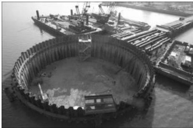
Figure 13. Cellular Cofferdam Breakwater project, Tuban. Indonesia (2005 – 2006)
