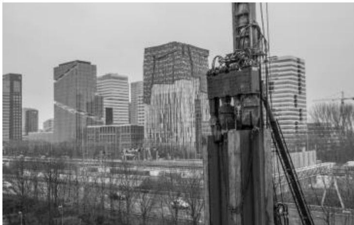
Figure 7. Phase 1 – Installation of Sheet Piles
