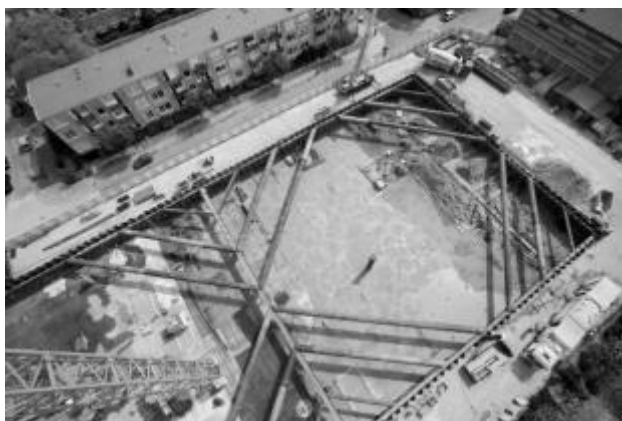
Figure 4. Plan View – Strutting system – During construction
