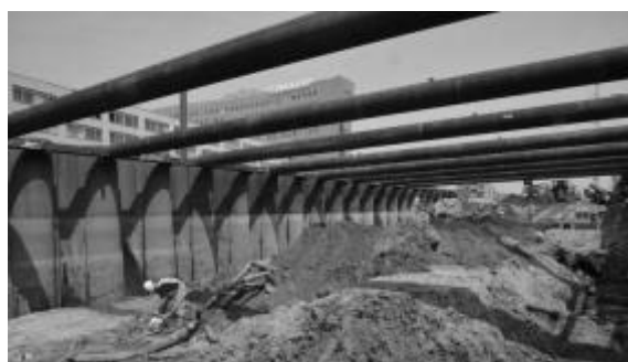
Figure 8. First row of Struts – Installation
